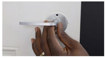
Place the lever side of the handleset to the interior side of the door with the handle end aligning into the hub of Panolock+.
