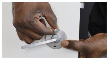
Secure the plates using the machine screws provided.
