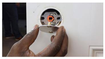
Align the exterior handset on the outside of the door panel. The screw bosses should be to the inside of the of the bore.
