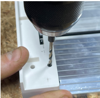
Using the jamb boot as the template, drill a 5/32" hole in the sill through the inner most hole. (use both holes for 6-9/16" jamb boot)
