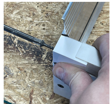
Attach jamb to the jamb boot with #8 x 1-1/2" screws. (Use three for 6-9/16" jamb boot.)
