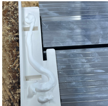
A. Caulk the top surface of the jamb boot.
