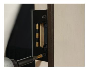
Secure assembly with two short screws provided, through strike plate.
