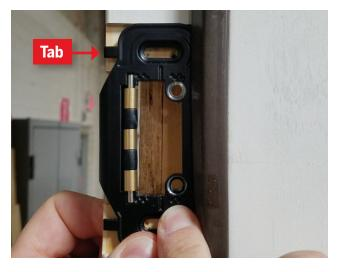
Place reinforcing roller plate into frame mortise. Orient tabs toward edge of frame. Align end of tabs with edge of frame.
