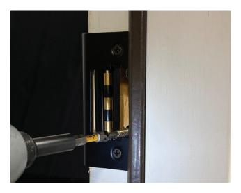
Place two long screws provided, through holes in reinforcing roller plate.
