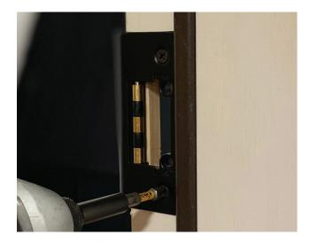
Retighten short screws to secure strike plate assembly at its adjusted position.
