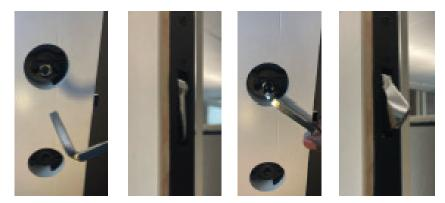
Insert construction handle into the handle-set location to check operation of the center latch. The handle-set will only affect the center latch, not the upper and lower tapered bolts.
