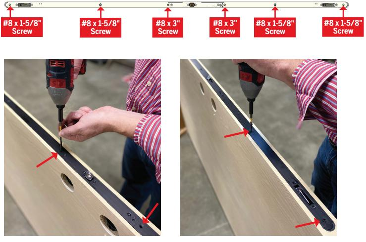
**Two #8 x 3" Screws:** Place through open holes just above the latch, and just below the spring adjuster screw.
