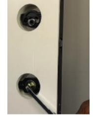
Insert construction handle into the handle-set location to check operation of the center latch. The handle-set will only effect the center latch, not the upper and lower latches.
