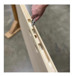
Ensure lock mortise in panel edge is clear of dust and debris.
