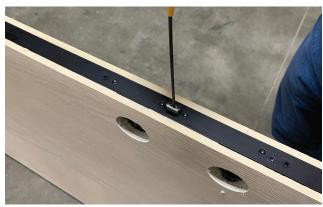
Tighten screw to secure latch in place.
