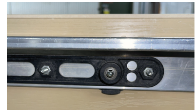
Handleset bore with rail attached and pin inserted
