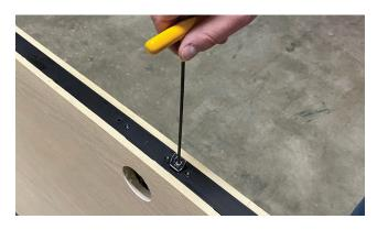
To rehand the lock, loosen the latch screw with a 9/64" allen wrench.
