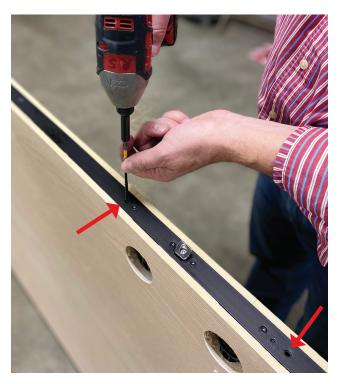
**Two #8 x 3" Screws:** Place through open holes just above the latch, and just below the spring adjuster screw.
