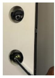
Insert construction handle into the handle-set location to check operation of the center latch. The handle-set will only effect the center latch, not the upper and lower latches.
