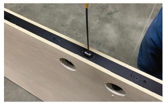
Tighten screw to secure latch in place.
