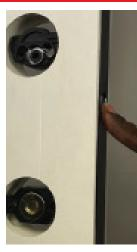
The center latch should easily go into the door panel when pushed with finger, returning to normal position when finger is taken away from the latch.
