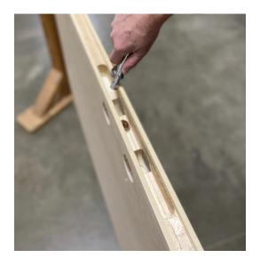
Ensure lock mortise in panel edge is clear of dust and debris.
