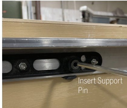
Handleset bore with rail attached
