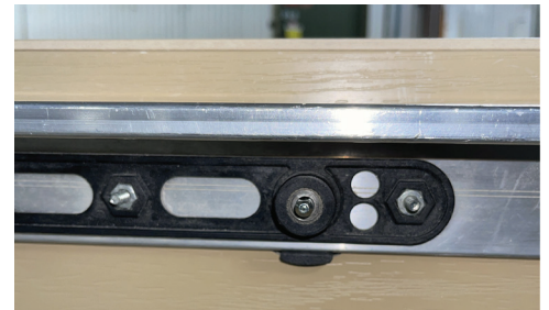
Handleset bore with rail and support pin in place
