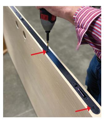
**Four #8 x 1-5/8" Screws:** Place through remaining open holes.
