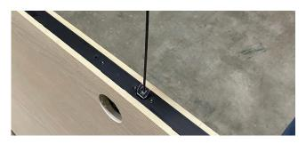
To rehand the lock, loosen the latch screw with a 9/64" allen wrench.
