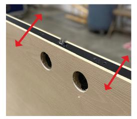
Check to confirm proper placement of the lock. Ensure entire length lock face plate is flush with edge face of panel. If lock does not sit flush, remove lock and check for debris in pocket. It may be necessary to verify mortise pocket dimensions if no debris or contamination is present.
