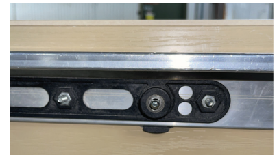
Handleset bore with rail attached and pin inserted
