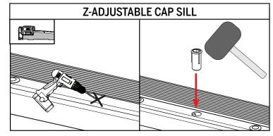
**d.** At the marked location on the sill, drill a hole **5/8" in diameter** and at least **1-3/8" deep.** Install the lower bolt receiver by tapping into the sill using a rubber mallet.
