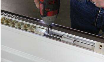
Now that the top of the astragal is secured, locate the pre-measured holes for each 1" screw, working from the top of the body of the astragal to the bottom.
