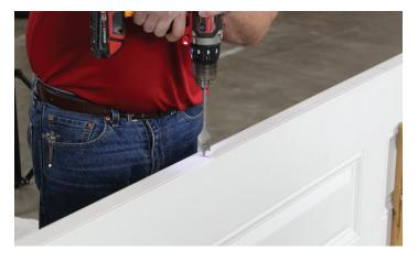
Once you've determined the locations for each latch, drill 1/2" deep into the center, top, and bottom marks with a 1" spade bit to create the latch bores.
