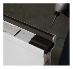
The last two screws should be secured under the sleeve covering the bolt on the bottom of the astragal. Remove the screw retaining the lower bolt sleeve, then gently remove the sleeve from the bottom edge to reveal the location for the two final screws.
