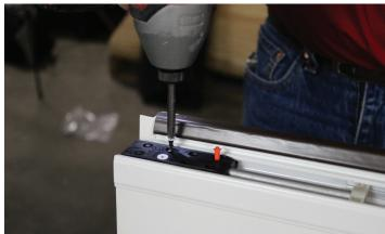
Taking care not to over tighten the screws, secure the two included 1.5/8" screws as close to the top edge of the astragal as possible, using the set of 4 predrilled holes in the plastic sleeve at the top of the astragal as a guide.
