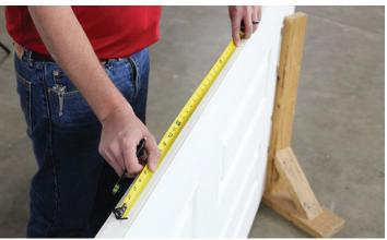
For 6'8 Doors: Measure up 28" from the center latch. For 8'0 Doors: Measure up 42" above the center latch.
