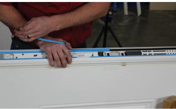
Leaving the adhesive backing in place, place the astragal on the door panel, making sure the top and bottom edges of the astragal are flush with the top and bottom edges of the door panel.
