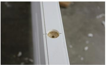
Clear the debris from the door panel prior to proceeding with the next step to be sure that debris doesn't get trapped between the astragal and the door panel and hinder installation or operation.
