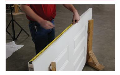
Measure to the latch height according to your door specifications and add 3 1/2".
