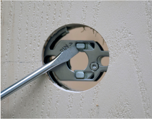
Move the pin button back to the starting position to disengage the upper, lower, and center latches.
