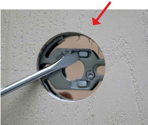
Use the screwdriver to push the pin to the right. The latch should fully retract.
