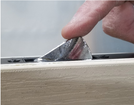
Push down on either of the multipoint latches. The latch should remain extended.
