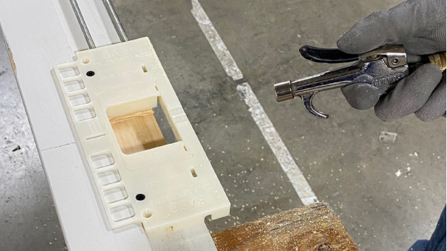
Turn router on. Rotate bit into center of template pocket to prevent damaging edge of template. Remove all material within template pocket. Remove all dust and debris from frame.
