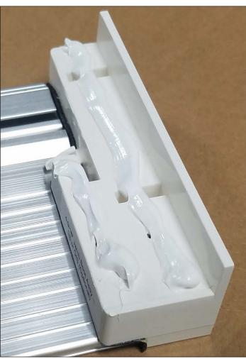
**D.** Caulk the top surface of the jamb boot, then align and place jamb on boot.
