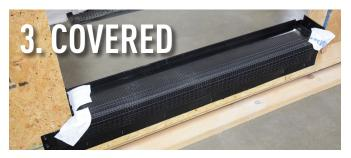
Fully seal corners with provided flashing tape and rest assured – you're covered.
