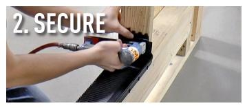
Place the sill pan in the rough opening and secure it into place utilizing screws or staples.
