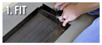
Cut and mold VersaPan using the built-in measurement markers to properly fit within rough opening.
