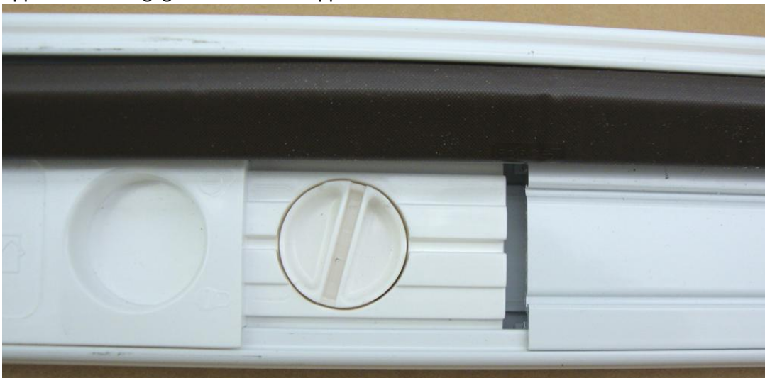
Upper Bolt Disengaged from Strike Support
