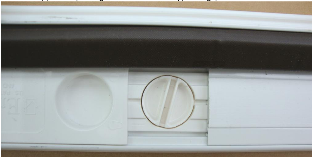
Bottom of Upper Bolt (Locking Knob Clears Strike Support Edge)
